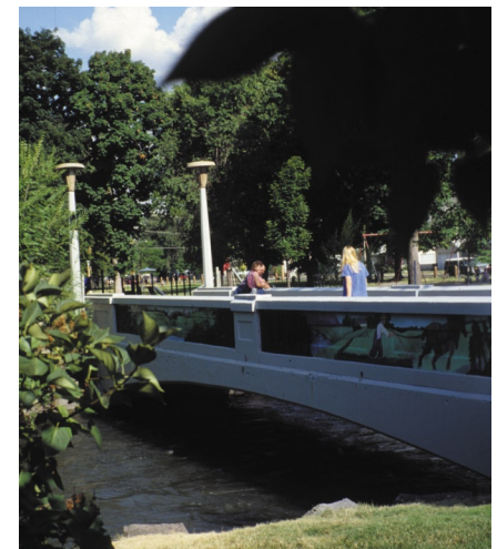
Bas relief murals on the sides of several old bridges along the parkway depict “the voice of the river” and stories from Baker City's Rich History. Photo: NPS-RTCA
